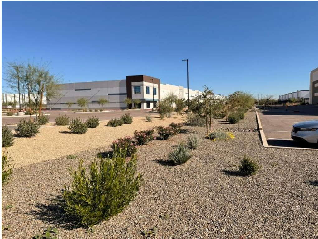
Figure 12. Northern adjoining industrial building.
