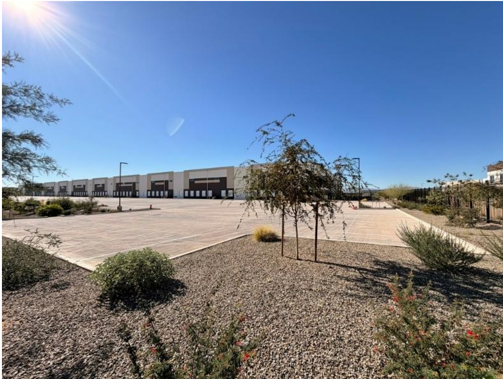
Figure 6. View of Property from northeastern corner, facing southwest.
