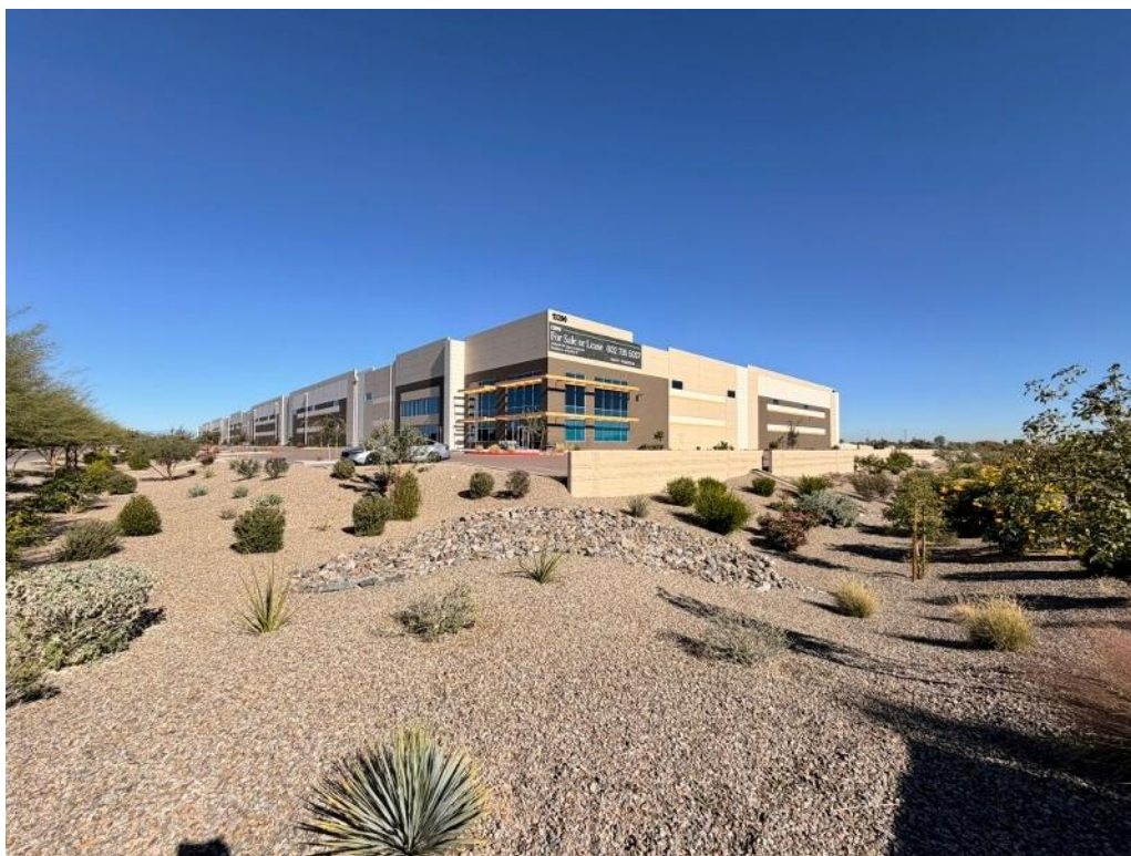
Figure 7. View of Property from southwestern corner, facing northeast.
