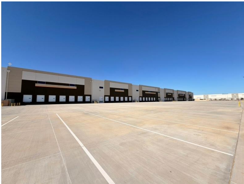
Figure 9. Eastern elevation, facing north.
